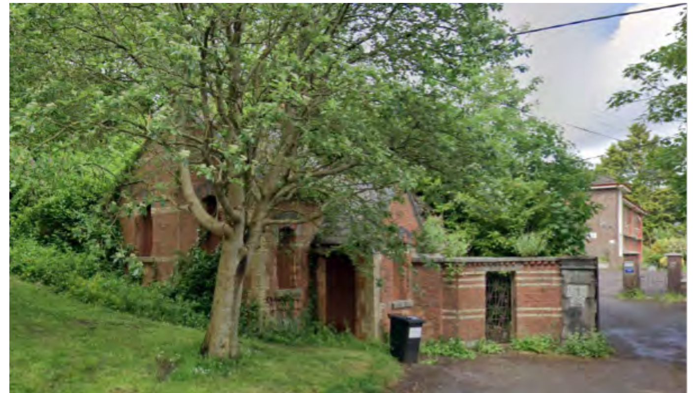
Figure 2.3 Gate Lodge (in foreground) and Former Hostel (in background). Image Source: Google Streetview
