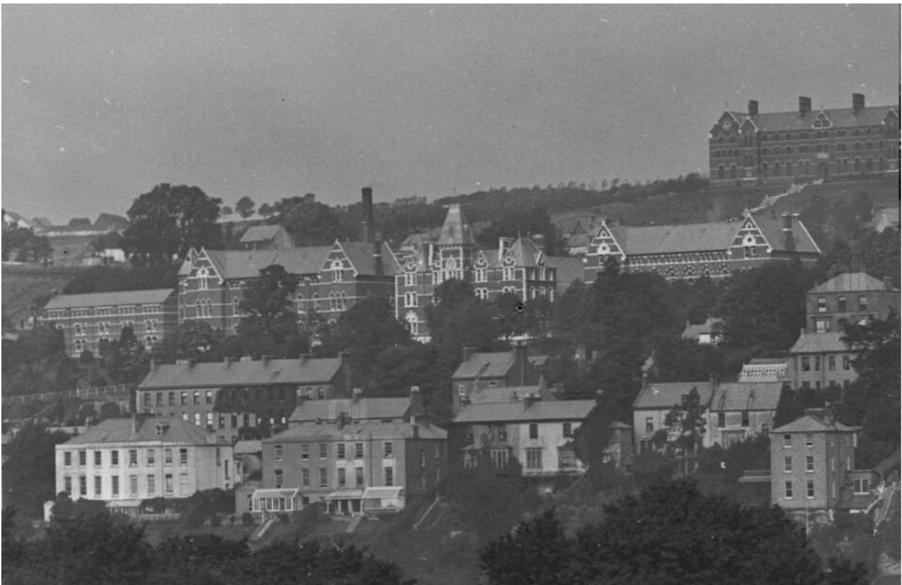
Figure 15.5: Post 1894 photograph of the Good Shepherd showing the recently constructed dormitory (and probably probationary home, completed by 1889). (NLI)
