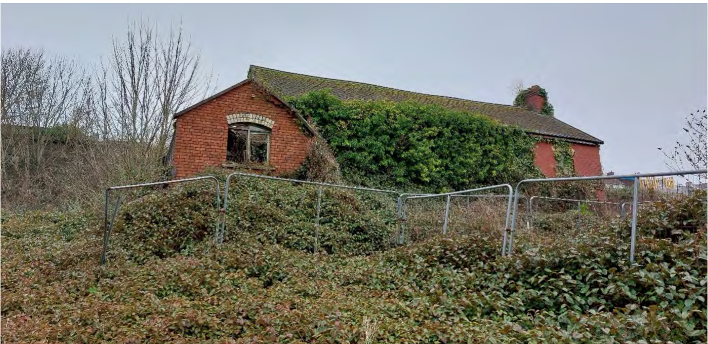
Figure 2.7 Bake House and Coach House. Image Source: Site Visit in February 2025
